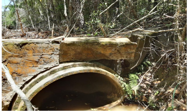
Headwall damage
