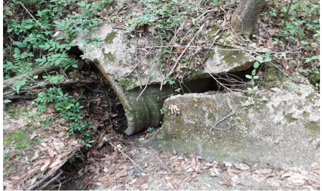
Headwall damage
