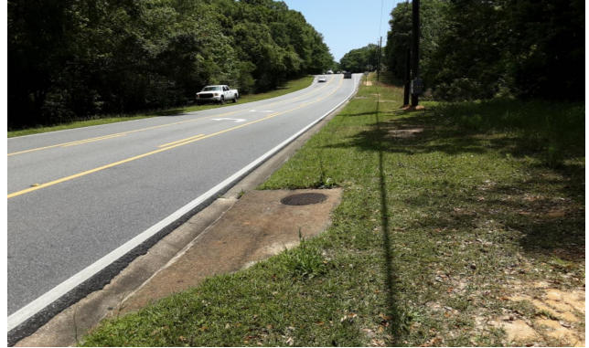
Measured pipe from this inlet
