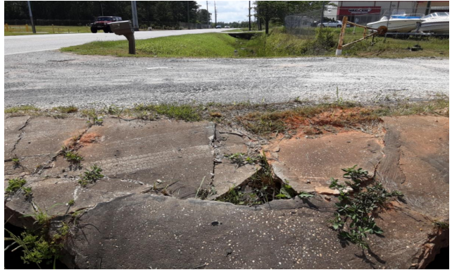
Headwall damage
