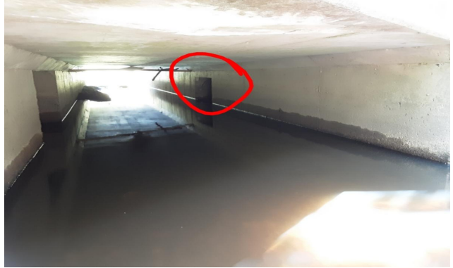
Outfall under road
