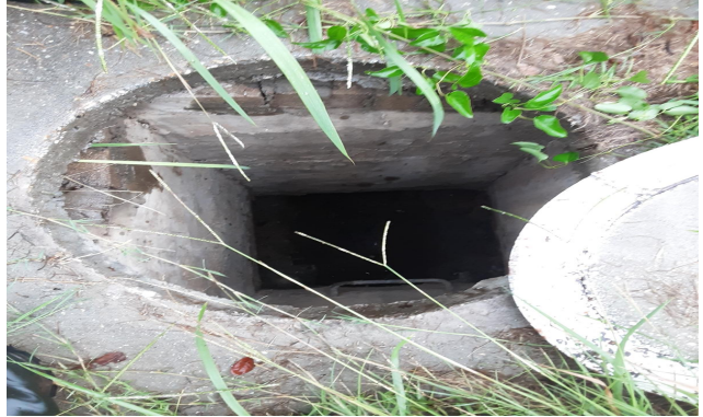
36 inch inlet junction box across street
