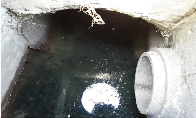
At inlet upstream of outfall
