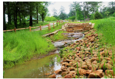
Gwinnett County, GA Regenerative Stormwater Conveyance at Ronald Reagan Park
