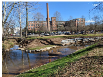
Greenville County, SC Brushy Creek Stream Restoration BMP Demonstration Project
