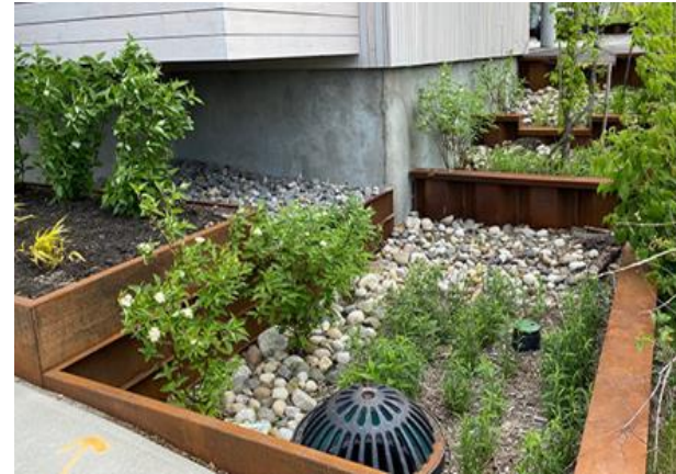
FocalPoint Modular Biofiltration System by ACF Environmental
