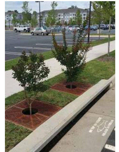
Filterra® Bioretention System by Contech® Engineered Solutions
