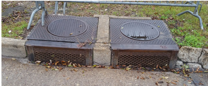
Figure 3-9 Catch Basin Screen Example
